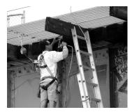
This NWCO wears a safety harness attached to a retractable lanyard system that would arrest a fall. This protection still provides enough mobility to install the bird netting on the bridge.
